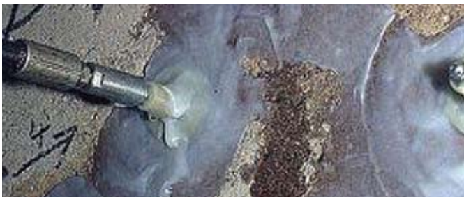
Epoxy injection for repair of crack
