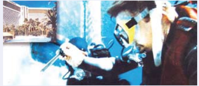
Hydrophobic foam injected in a basement pool
