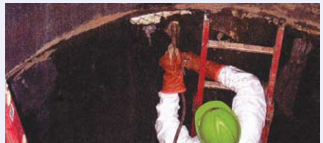
An injection specialist uses chemical grout to repair a leaking joint
