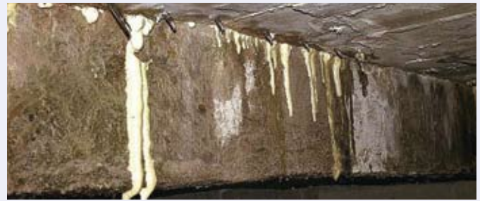
Hydrophilic expansive PU foam
