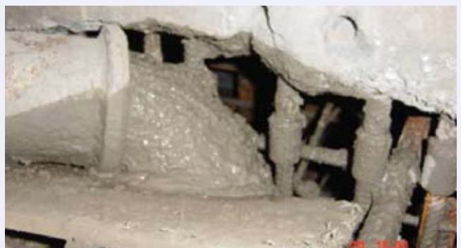
Figure: 4 Use of PCs in self-compacting concrete in Delhi Metro
