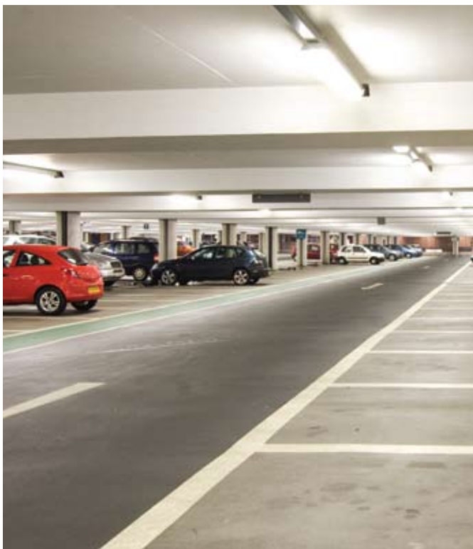
Figure 5 : Application of SRA Concrete in basement Parking
