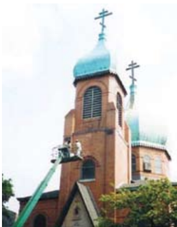
Fig 5: Cementitious crystalline waterproofing on external surfaces
