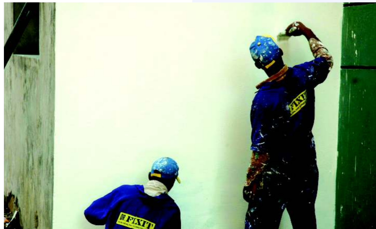
Fig. Application of high performance coating in progress
